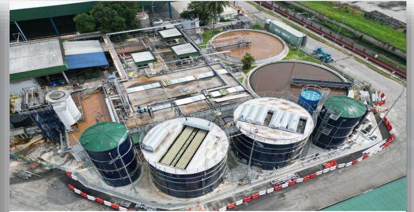
Wastewater treatment plant
