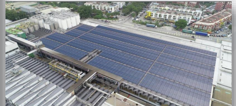
Solar PV on-site
